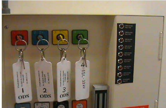
Mag-lock, Prox-entry Reader, EDR, EDR Re-set key, Switchgear Key-press and Issuer Keys
