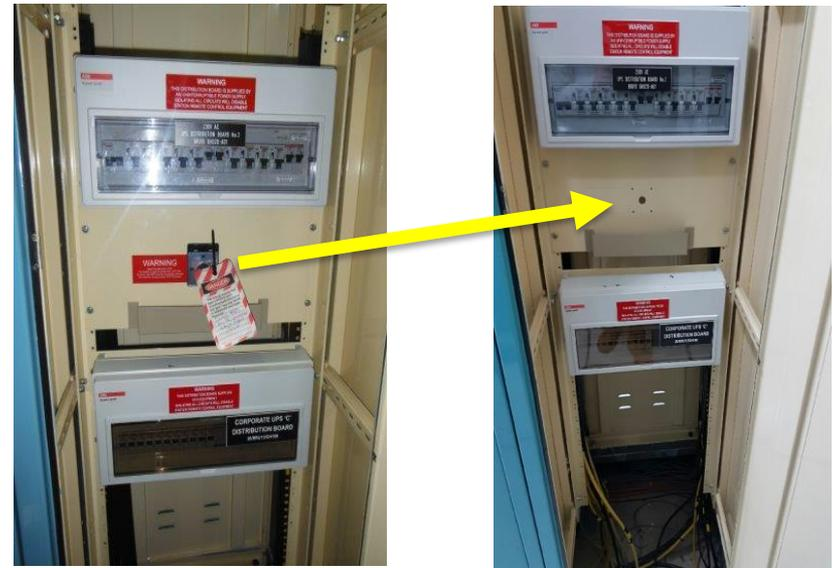
1. This switch allowed both DB's to be connected, to allow for one UPS to be taken out for maintenance while retaining both server pairs in service. A move to separate utilised power supplies required this functionality to be removed. The switch had been "tagged out of service" in the meantime to avoid operation.
