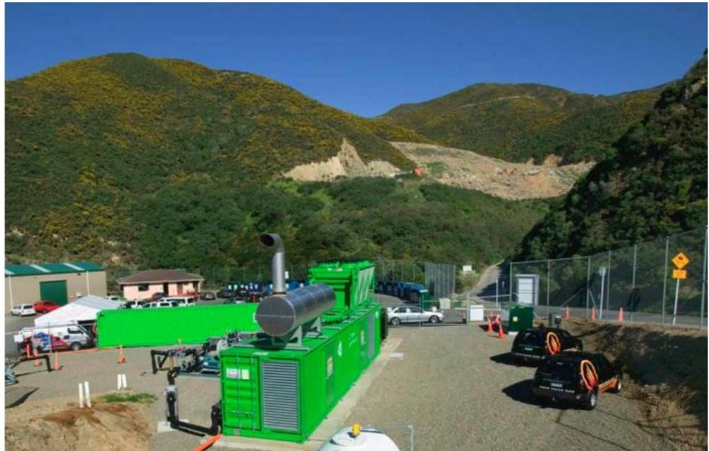
The Happy Valley landfill gas power plant is estimated to have cost NZ\$1,900 – 2,000/kW. However this specific capital cost includes a gas compressor skid, landfill gas piping, and provision for a further genset to be added in the future. When these features are deducted the specific capital cost is estimated to be NZ\$1,500/kW.
