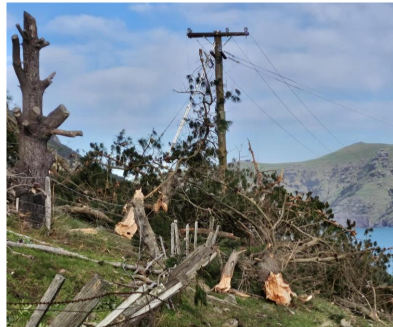
Fallen trees damage electricity lines, source: Electricity Networks Aotearoa
