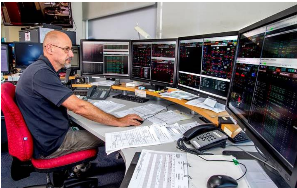
Vector's Network Control Room, Auckland
