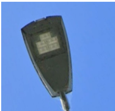
C1 SUPPLY AND INSTALL A GROUND PLANTED OCTAGONAL GALVANISED STEEL COLUMN WITH A 2M OUTREACH ARM (REFER TO SPECIFIC NOTES 'G' AND 'H' ON DRAWING DG-R-4301) COMPLETE WITH AN AEC ITALO 2 SV 4.5 5M 75W LED LUMINAIRE (8090 LUMENS). THE LUMINAIRE SHALL BE MOUNTED AT A HEIGHT OF 10M AND BE TILTED AT AN ANGLE OF 0° TO THE HORIZONTAL.
