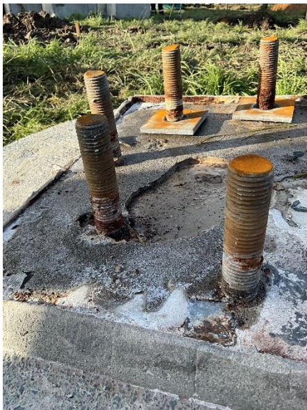
Photo A.5: Leg B foundation holding down bolts. No damage to bolt threads observed.
