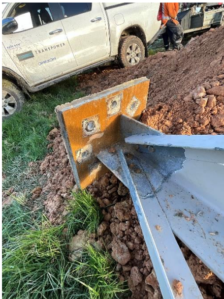
Photo A.21: Top side of leg C base plate. Sign of sand blasting, as shown by presence of surface rust on the top of the base plate and paint removed on the leg members.
