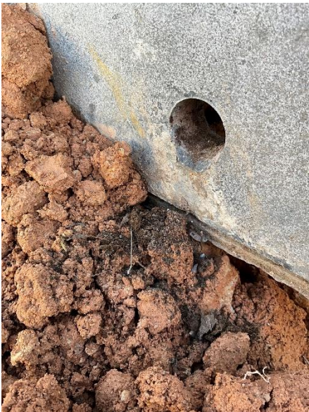
Photo A.20: Underside of baseplate of leg C. Some damage to the bolt hole closest to the ground (eastern side of base plate), which aligns with broken bolt.
