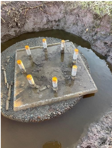
Photo A.3: Leg A foundation after being drained. No holding down bolts with nuts installed. No damage to bolt threads observed.
