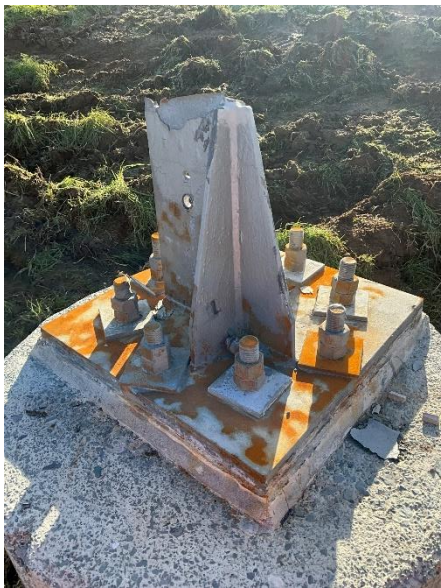
Photo A.14: Leg D ruptured. No nuts removed.
