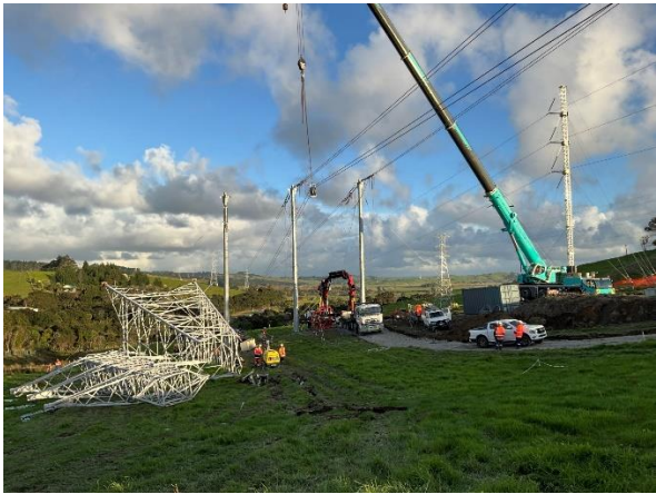
Photo A.1: Temporary restoration works. Western circuit supported by Lindsey tower (right), eastern circuit restoration using three steel monopoles in progress (middle), Tower 130 relocated from fallen location (left).
