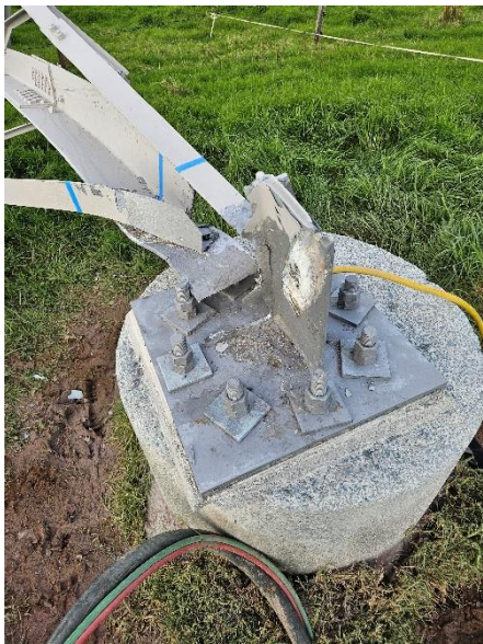
Photo B.9: Leg D ruptured leg and foundation.
