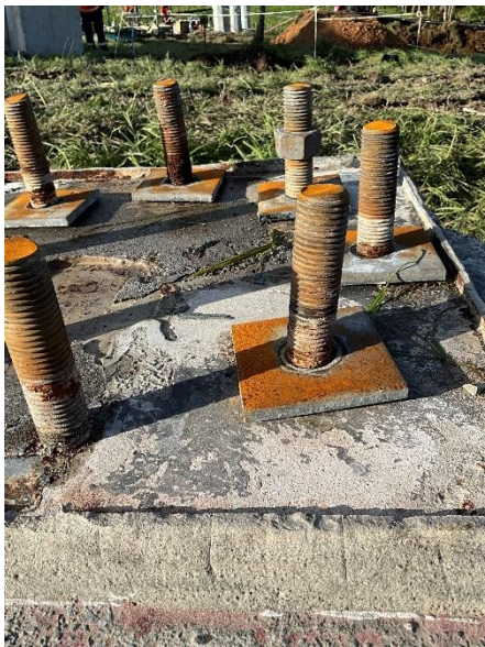
Photo A.6: Leg B foundation holding down bolts. No damage to bolt threads observed.
