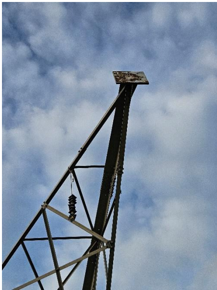
Photo B.11: Eight nuts and square washers tied with rope to leg A.
