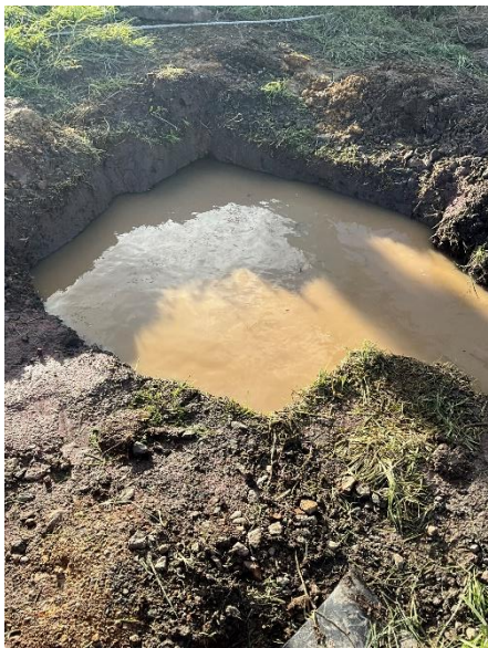
Photo A.7: Leg C foundation underwater upon arriving to site, prior to being drained.
