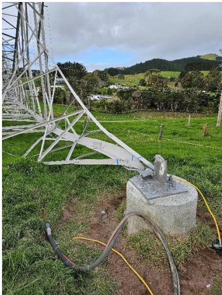
Photo B.8: Leg D ruptured leg and foundation.
