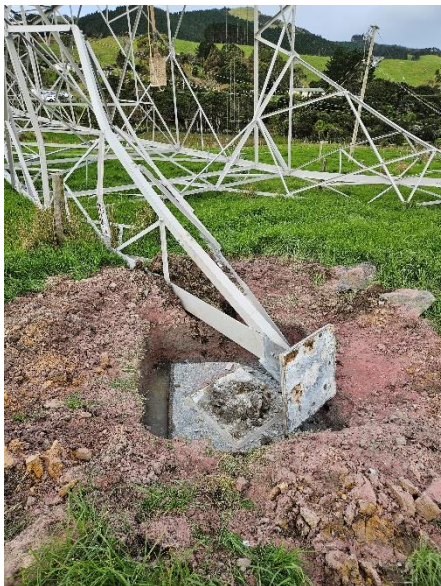
Photo B.6: Leg C leg and foundation.
