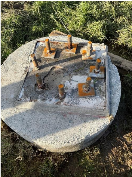
Photo A.4: Leg B foundation holding down bolts. Square washers and nut suspected to be placed back on bolts after tower fall. No damage to bolt threads observed.
