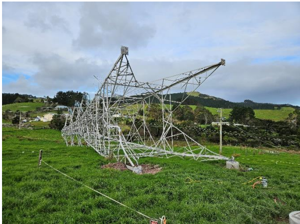
Photo B.2: Tower in the fallen location. Legs C and D are in close proximity to foundations indicating the tower fell square with the line in the transverse direction.
