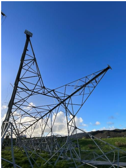
Photo A.16: Legs A and B of fallen tower (top of image). No obvious damage observed from ground level. Approx. 8 nuts and square washers tied via rope to leg A.
