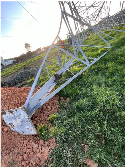
Photo A.18: Leg C of fallen tower. Damage to k-brace member.
