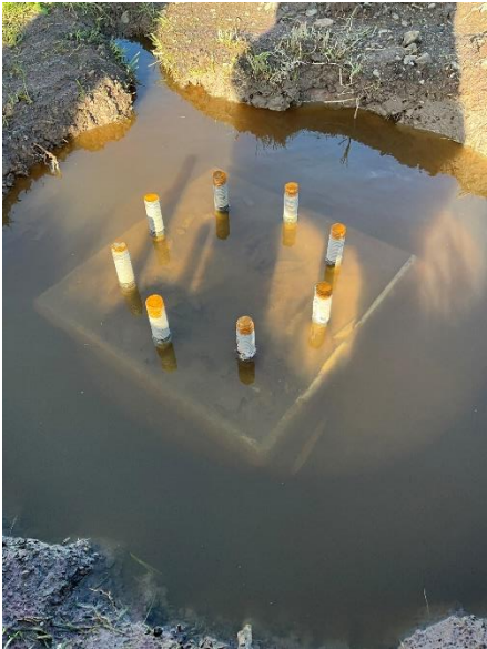
Photo A.2: Leg A foundation underwater upon arriving to site, prior to being drained.
